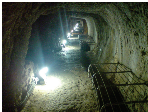
Abb. 6: Blick in den Tunnel
